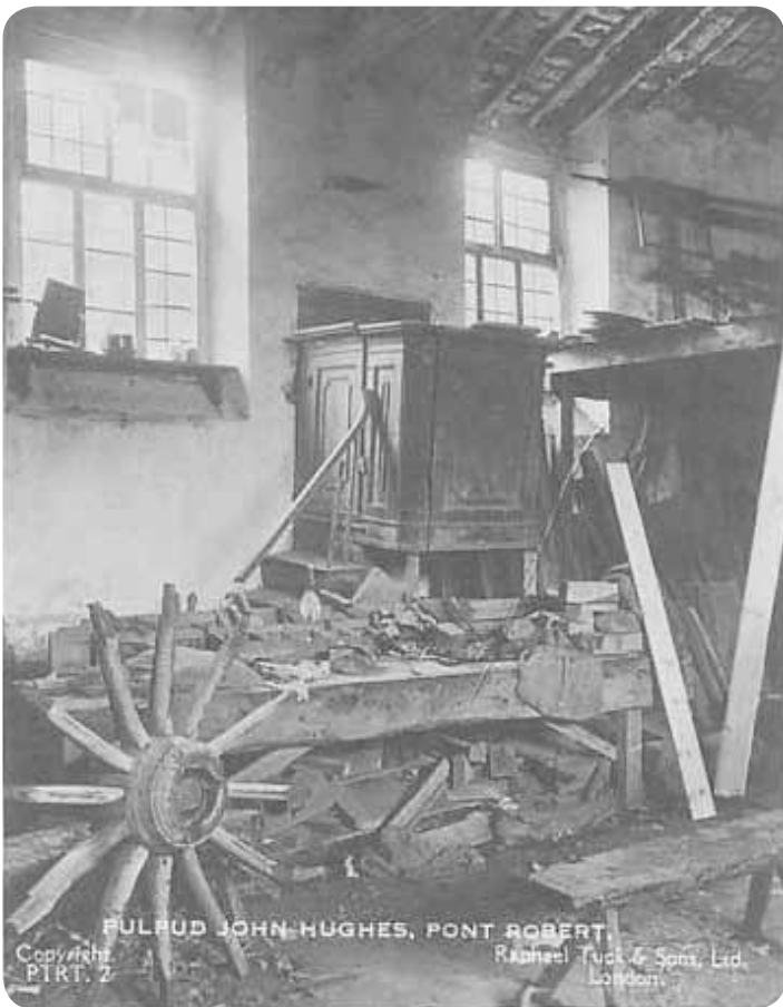
The neglected interior and the John Hughes pulpit before it was repaired. A clause in the deeds prevented its removal.
